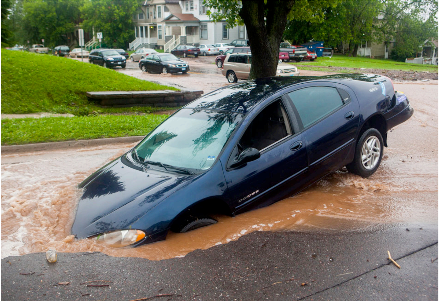
Duluth, Minn. — A sinkhole got the better of this car at the corner of First Street and Seventh Avenue East Wednesday morning after heavy rains caused flooding in Duluth, Minn. (Derek Montgomery for MPR) ( Read more about the flood ) LINK TO THIS PHOTO
