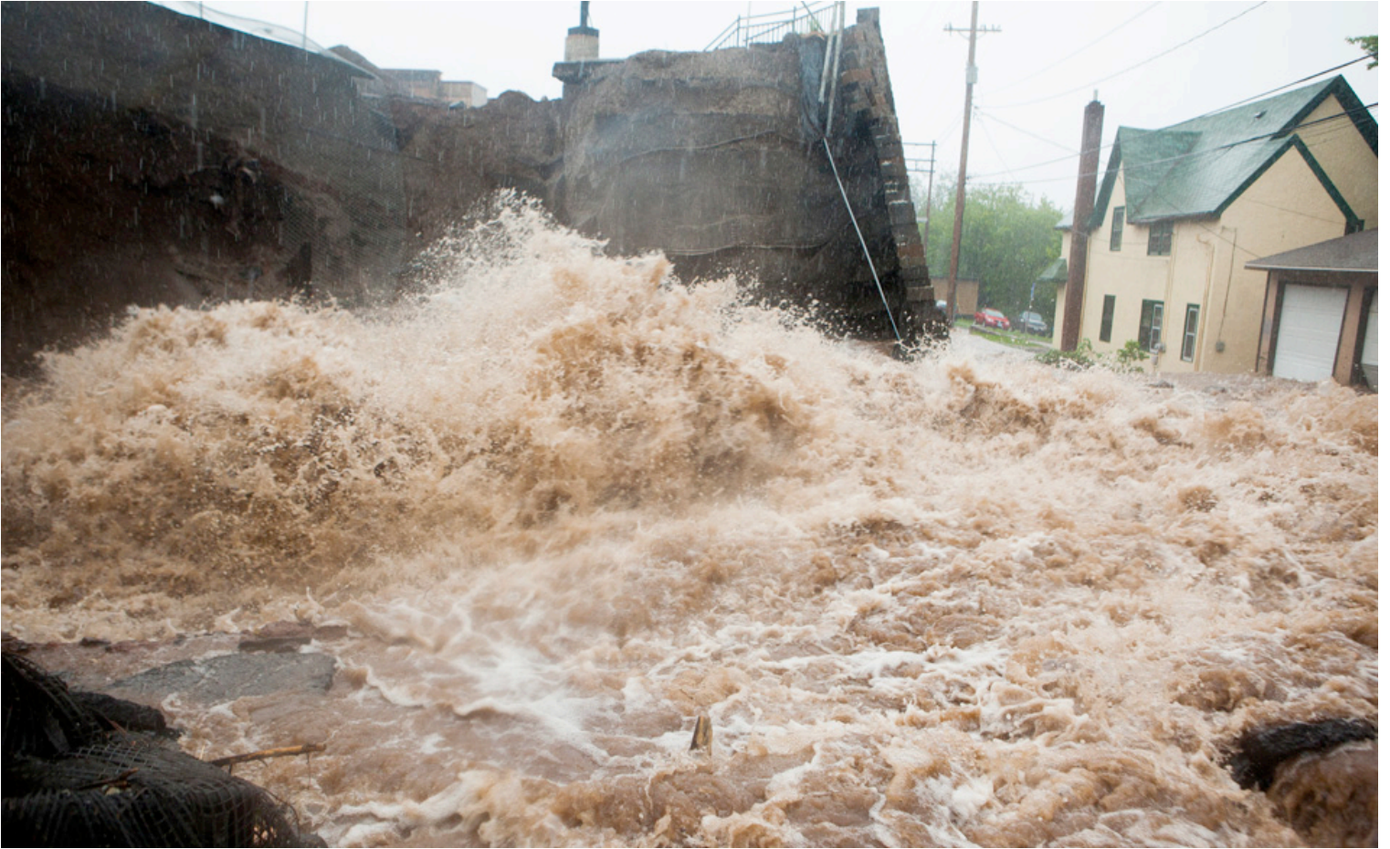
Duluth, Minn. — Brewery Creek burst through a retaining wall adjacent to the Whole Foods coop Wednesday morning after heavy rains caused flooding in Duluth, Minn. (Derek Montgomery for MPR) ( Read more about the flood ) LINK TO THIS PHOTO
