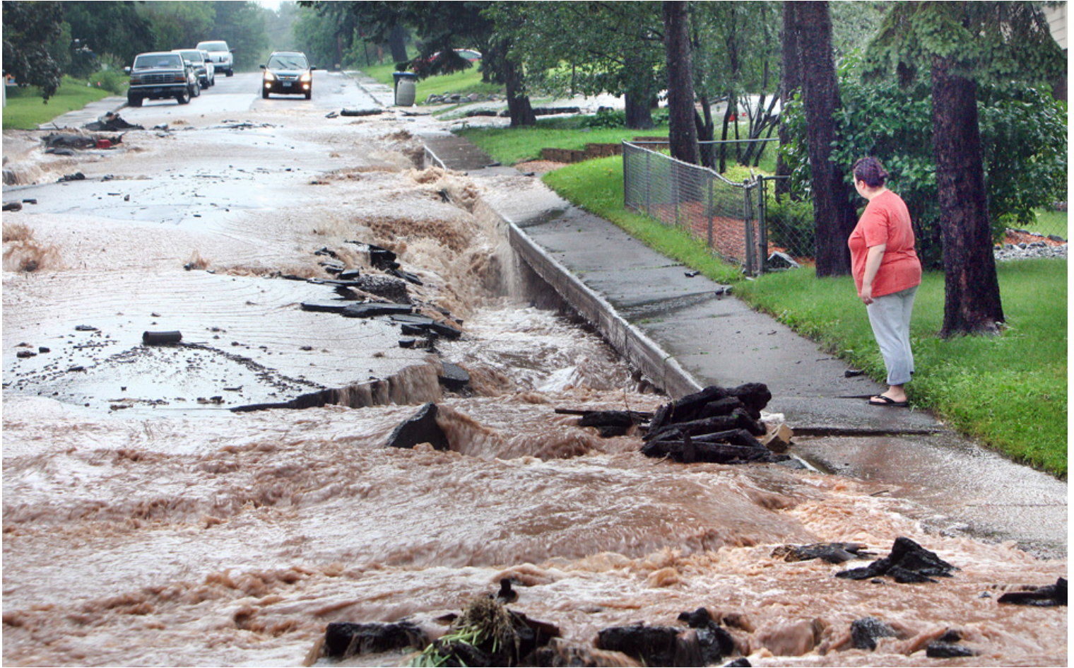
Duluth, MN, USA — Water flows down a damaged street in Duluth, Minn. on Wednesday, June 20, 2012. (AP Photo/The Duluth News-Tribune, Bob King) ( Read more about the flood ) LINK TO THIS PHOTO
